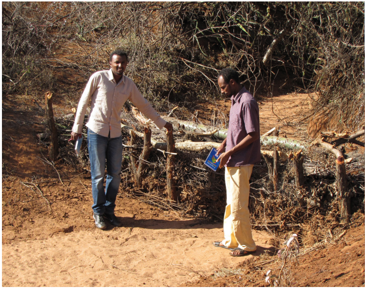
A pair of photos showing (left) an intact sieve structure and (right) the same structure destroyed by flooding in the heavy spring rains. All the branch packing, the large ballast logs, and most of the upright stubs have been washed away in the right photograph. (Photo credits: (left) Brien E. Norton and (right) Bedasa Eba).
