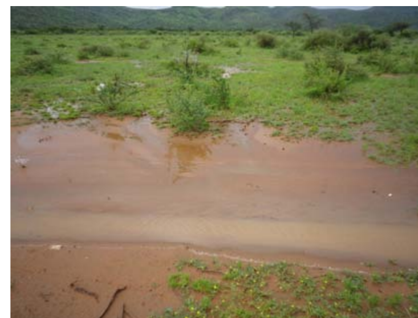
Figure 9. This is an example of how poorly located and constructed access tracks can drain landscapes as effectively as any true donga. In this case a creek from the mountains in the background has flooded out in a fan when it has hit flat ground, depositing rich alluvium in a highly productive system. The track is cut into the land and has started micro-terraces (broad, small water fall heads) cutting back into the floodout fan. The track starves areas of the fan below it.
